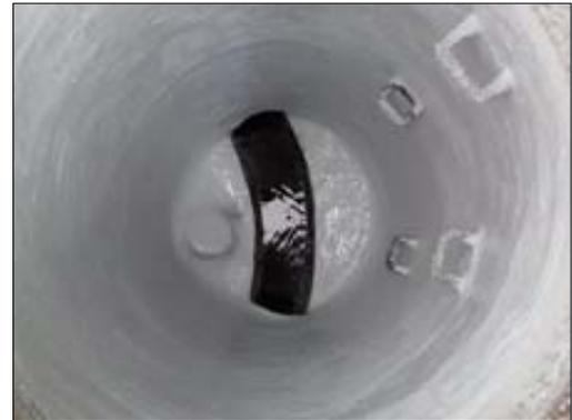
**MH LINER CEMENT MORTAR APPLICATION:** Thoroughly clean and remove any loose or foreign materials including paints, dirt, oil, grease, surface coatings, laitance and any other bond-inhibiting material from surface to be coated, using minimum 3500 psi waterblast. Stop all active leaks. (Please refer to our Manhole Rehabilitation Specifications for product selections.) Surface should be Saturated Surface Dry (SSD) just prior to material application. Any standing water must be removed.
