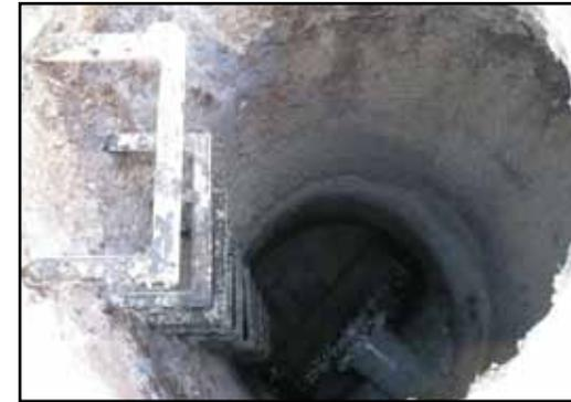
SEVERELY DETERIORATED, SEVEN YEAR OLD PUMP STATION DISCHARGE MANHOLE IN CENTRAL OHIO.
