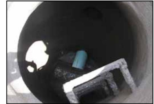
SAME MANHOLE AFTER REHAB WITH 1.5" THICK CEMENTITIOUS LINER WITH ANTIBACTERIAL ADDITIVE.
